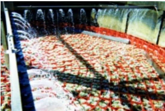
Plastic straws recovered from returnable bottles are used to filter wastewater as part of a progressive water-management program where the employees initiate the solutions.
