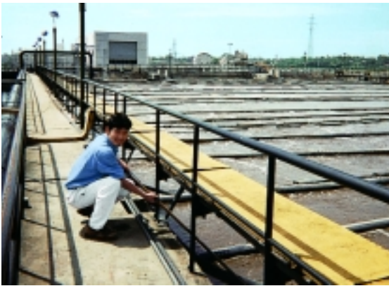
Budweiser-Wuhan International Brewery's investment in wastewater treatment technology helped reduce by 50 percent the quantity of waste solids for disposal.
